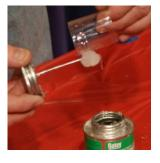
Wipe off any glue that squeezes out between the two fittings. The two fittings should fit tightly together.
